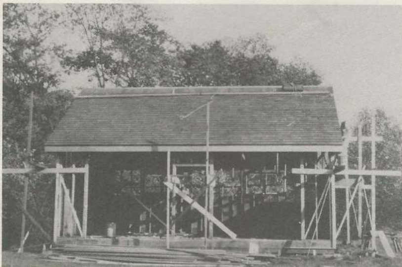
Building the Quartermaster Lodge — 1931.
